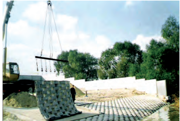
Flexible apron works
