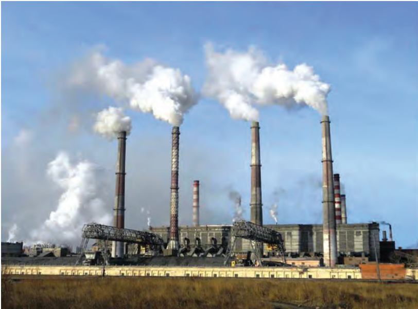
Flue gas purification
