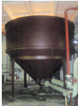
Protection from corrosion: internal and external areas of filter pipes (left); H-cationite filter reservoir (central); and demineralized water tank (right)
