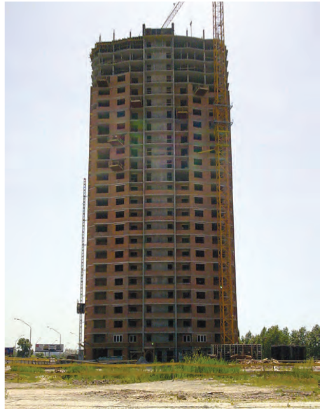
27-floor house at Obolonskiy Avenue in Kyiv with shock isolation system (situated in 100 m from shallow subway line)
