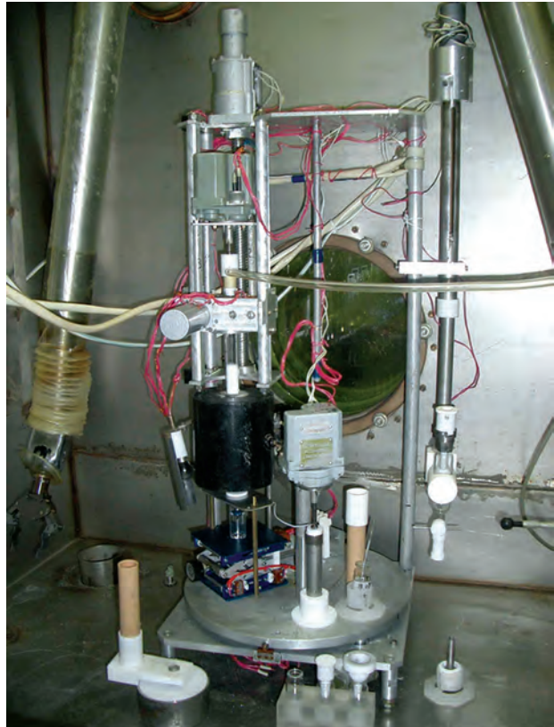
Plant for production of sodium iodide ( 131 I) capsules
