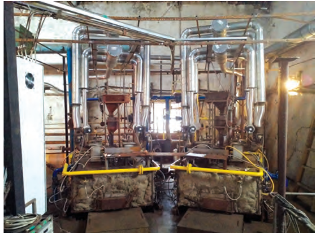
General view of the plant
