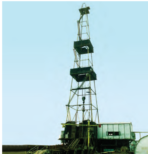
Derrick at well No. 8
