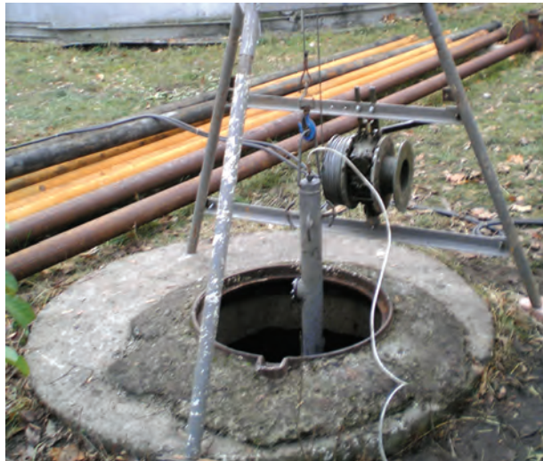
Debit recovery of water supply well No. 3754 located in Irpin
