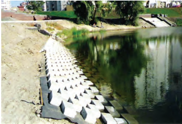
Flexible apron of Pozniaky pond banks with the use of Texivod
