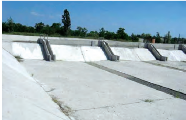
Rehabilitated sludge bed
