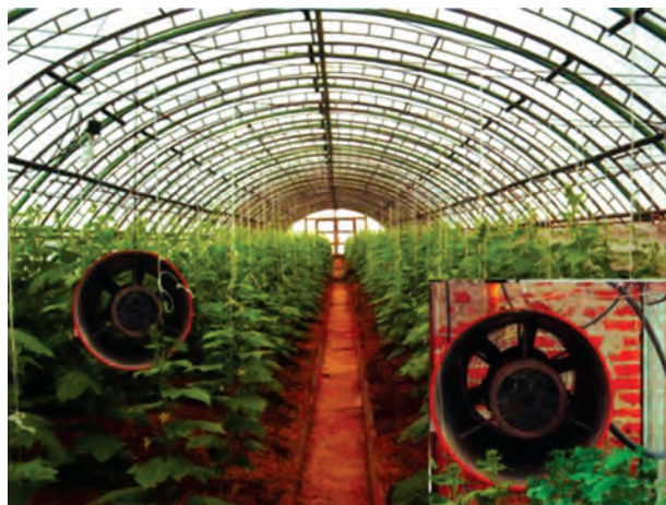
Catalytic heat generators (CHG), combustion chamber of gas turbine
