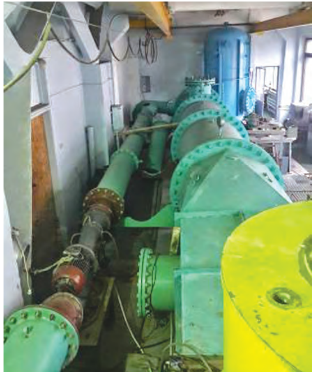
Installation for testing micro-HPP on the ECS-30 stand
