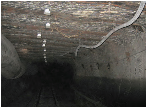
Roof-bolting support scheme
