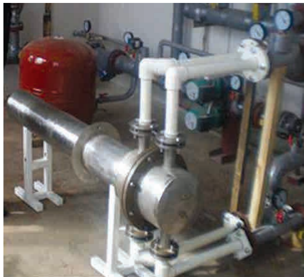
Heat exchanger mounted and installed
