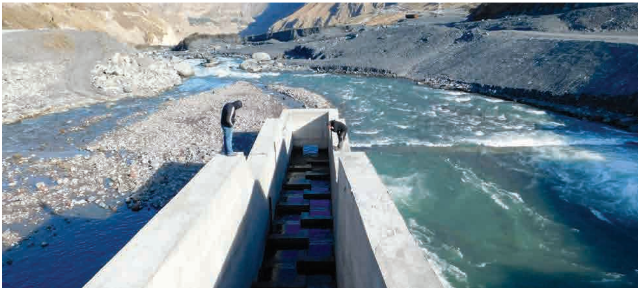
Fish-pass facility on the Terek River (Georgia) built designed by the Institute of Hydrobiology
