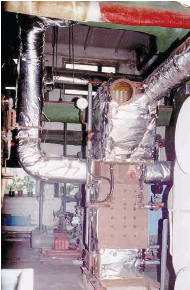
Heat-recovery exchanger BAP-1.5 behind the boiler with a heating capacity of 0.63 MW
