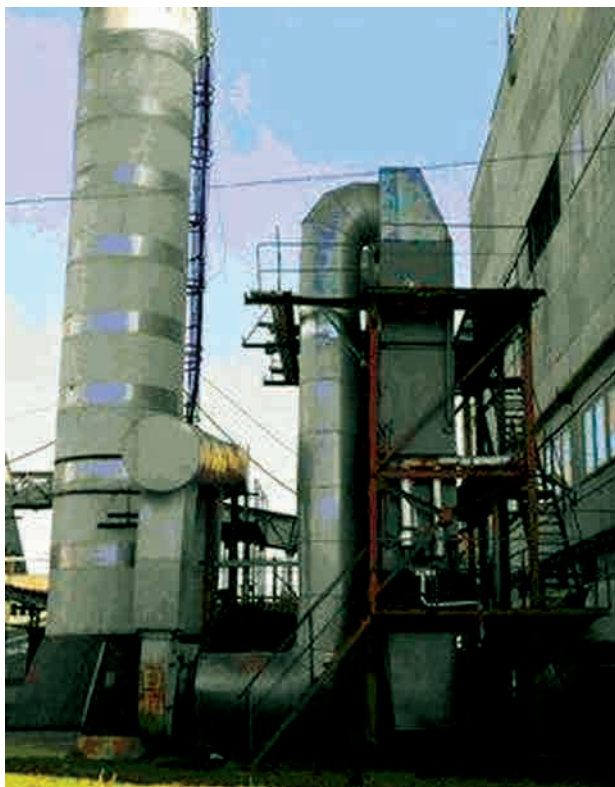
MWH heat-recovery exchanger for glass furnace
