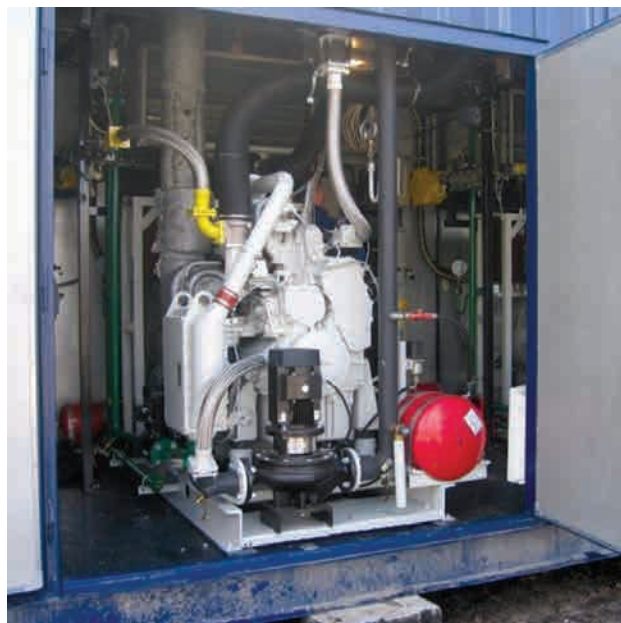
Gas power plant based on an internal combustion engine with a capacity of 185 kW
