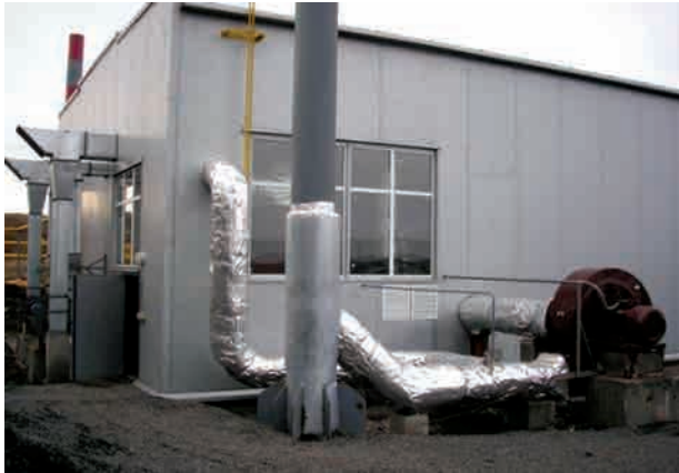
Garage defroster for simultaneous defrosting of ore in 12 railway cars
