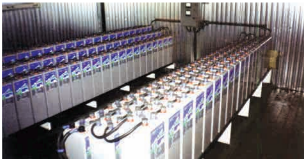
Electrical storage system of the station
