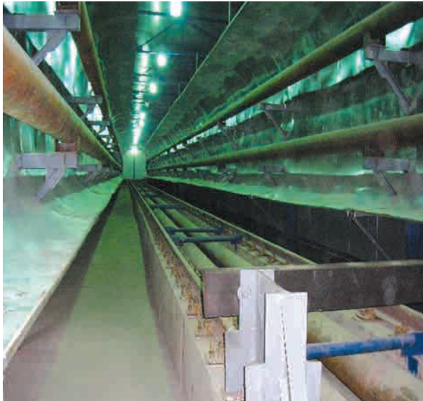
The garage defroster interior with radiant pipes and screens
