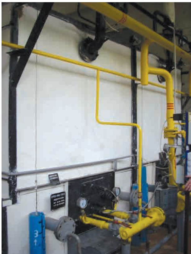
Mounted hearth burners in NDISTU-5 boiler
