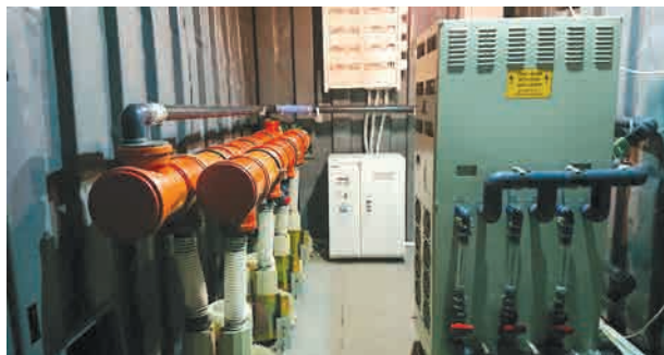
Ozone system for treatment of agricultural disperse products based on Stream Ozone OzW50 (up to 100 gO 3 /h) ozone generator
