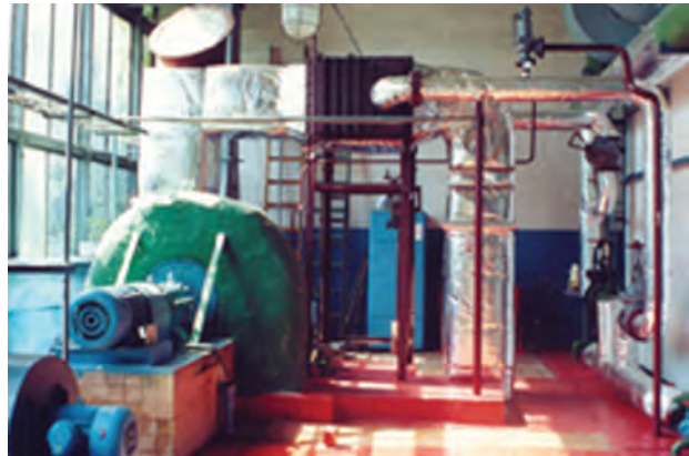
Heat recovery plant with convection bank PK-1-102 sh installed behind TVG-4r boiler at the boiler house at 2a Osipovska St., Kyiv
