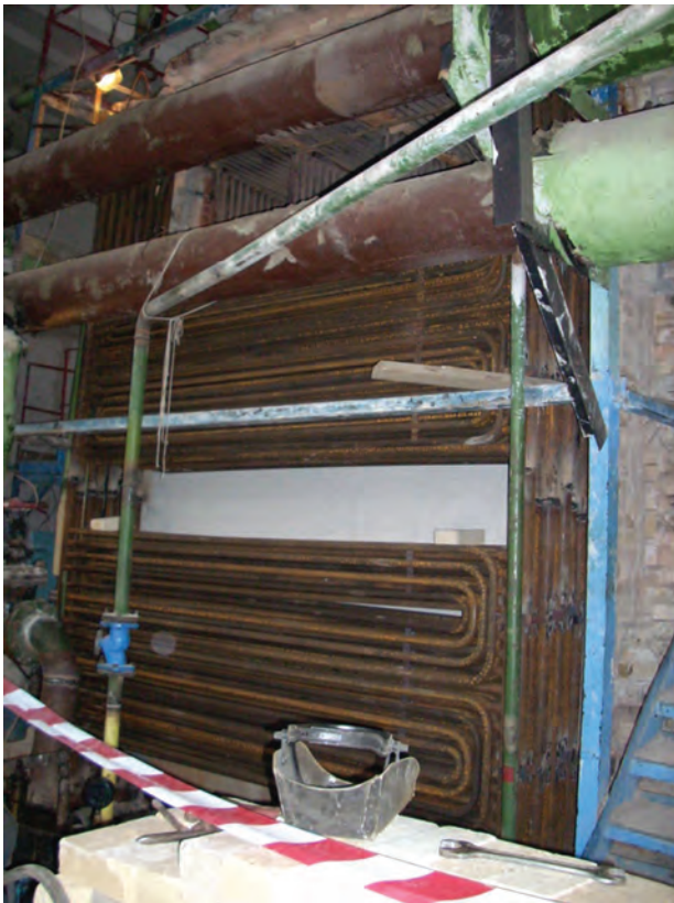
◀ Installation of convective surface made of \text{Ø}32 \times 3 mm pipe instead of original \text{Ø}28 \times 3 mm one in TVG-8M boiler
