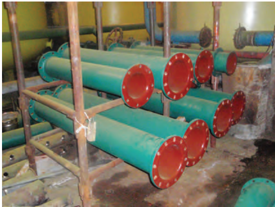
Protection from corrosion: internal and external areas of filter pipes (left); H-cationite filter reservoir (central); and demineralized water tank (right)
