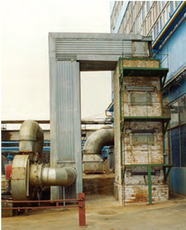
Heat recovery plant with TVM regenerator installed behind the furnace No. 3 of Hostomel Glassworks in Kyiv Oblast
