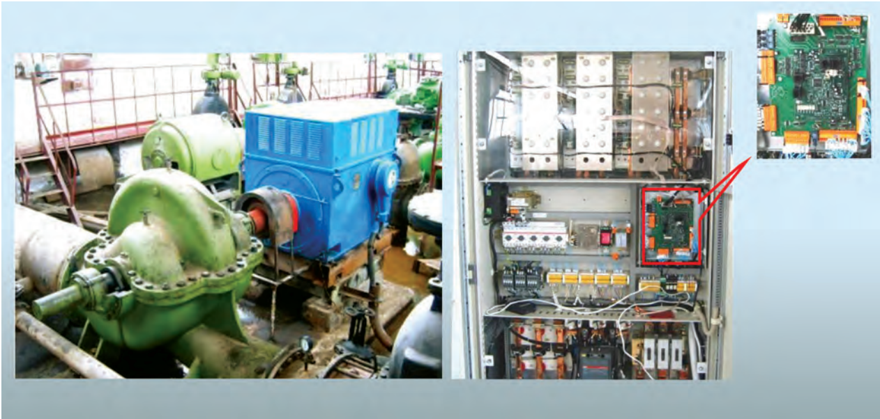
Adjustable electric drive of 750 kW pump based on doubly-fed electric machine
