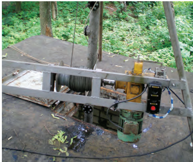
Debit recovery of water supply well No. 3754 located in Bucha
