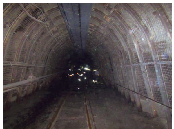
The stability of a mine working with the frame anchoring system during mining operations in the zone of high-amplitude geological disturbances
